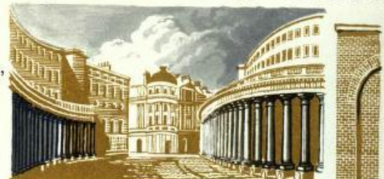
A The Quadrant, Regent Street 1818 Cast-iron columns
